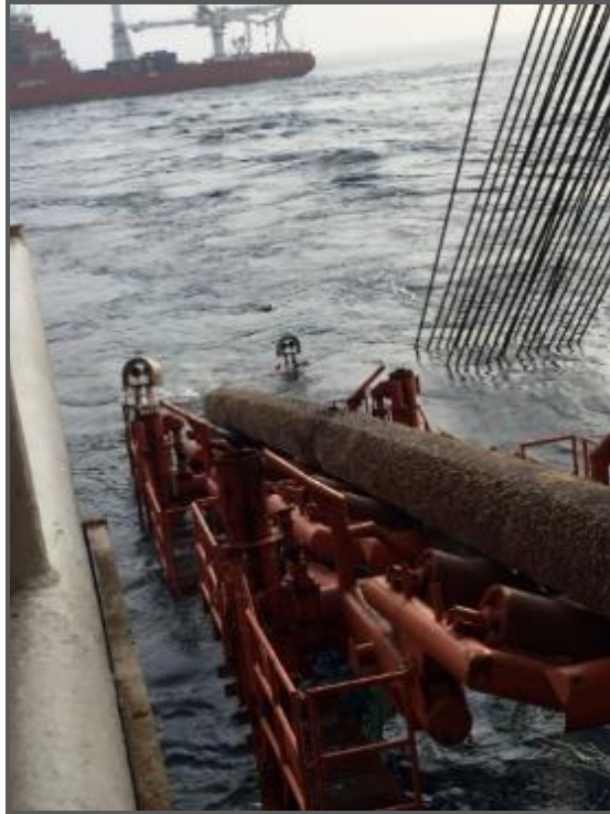
Figure 8: Pipeline recovered to lay barge
