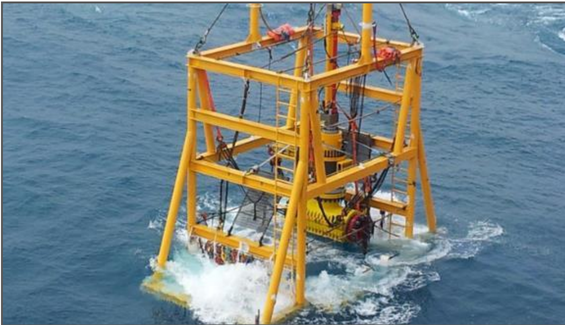
Figure 4: Mechanical clamp and hot tap machine deployment
