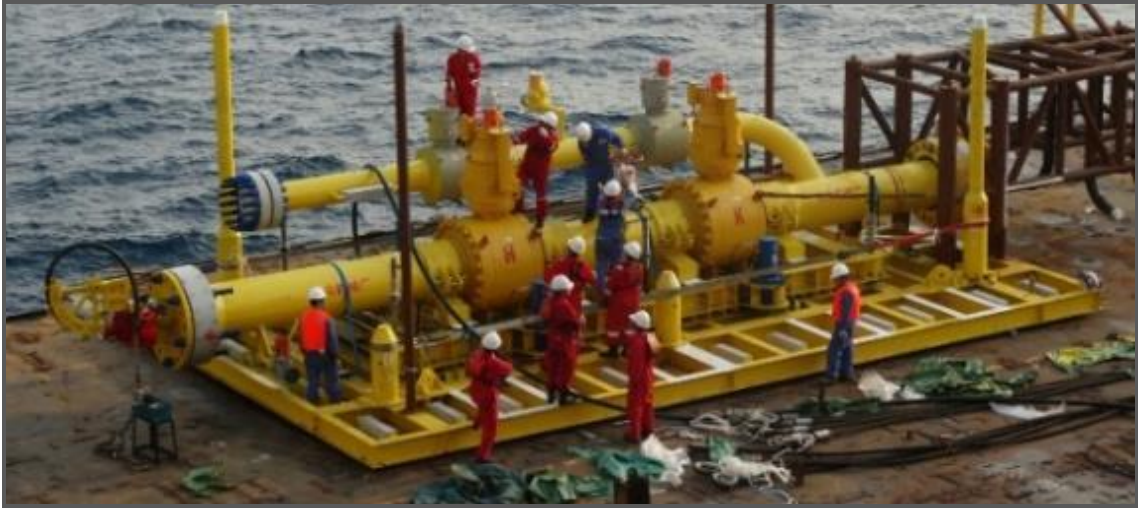
Figure 9: Pipeline End Manifold (PLEM) deployment
