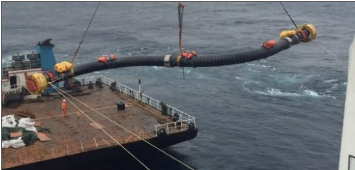
Figure 10: 25m tie-in spool deployment
