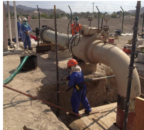
Tecno Plug deployment system in temporary launcher
