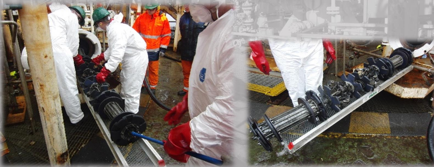
Receive of bi-directional GEO+ inspection tool in 2013 execution
