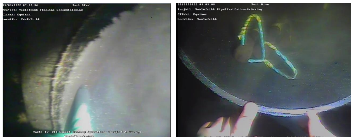
Figure 8. Pictures from the diver show the clean pipe wall.
