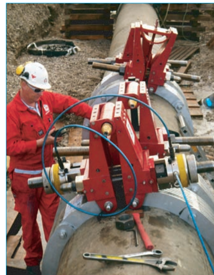
Fig.3. Mounting the tension belts onto the pipeline.
