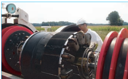
Fig.1. One of the 38-in SmartPlug trains on its way into the launcher.
