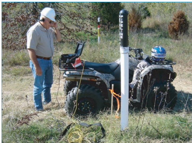
Pig tracking in progress.
