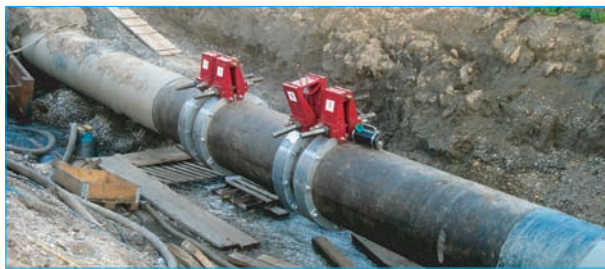
Fig.2. The SmartPlug train is situated just below the custom-made tension belts. The pipeline contains gas with a pressure of 50bar held back by the plug train while work continues safely to connect to the new pipeline.
