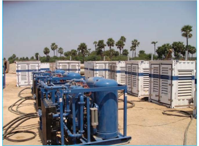
BJ's spread used on the RGTIL project.
