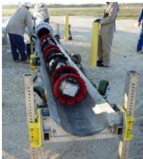
TDW deploys EMAT inspection
