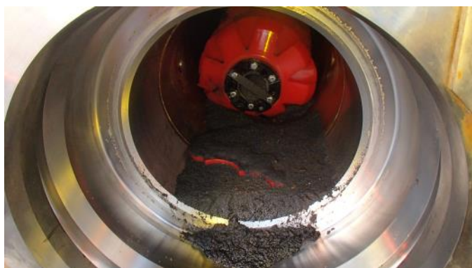
De-sanding pig and debris in receiver during operational cleaning
