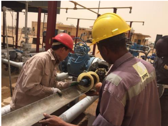
Geometric pig launching at worksite
