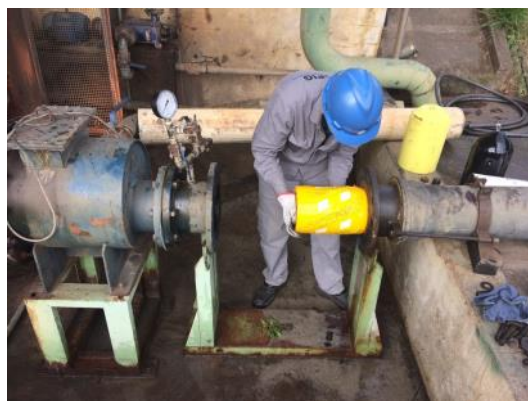
Cleaning pig installation point
