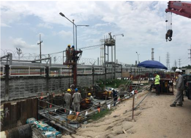
Worksite photo in Thailand ●
