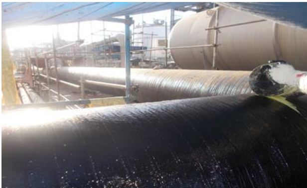
Elbow reinforcement – R4D wrapping on progress ●
