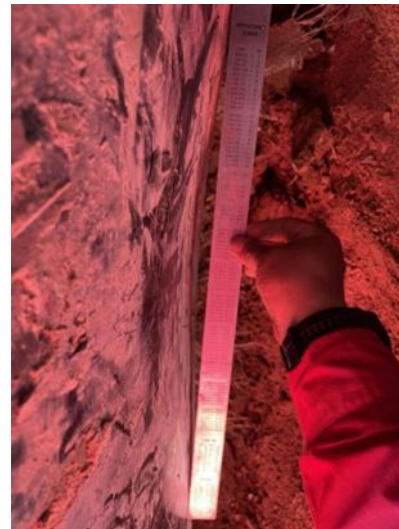
Photo of excavation
