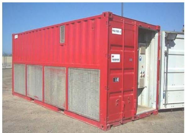
Figure 8: P&SS Sirocco<sup>SM</sup> air drying unit
