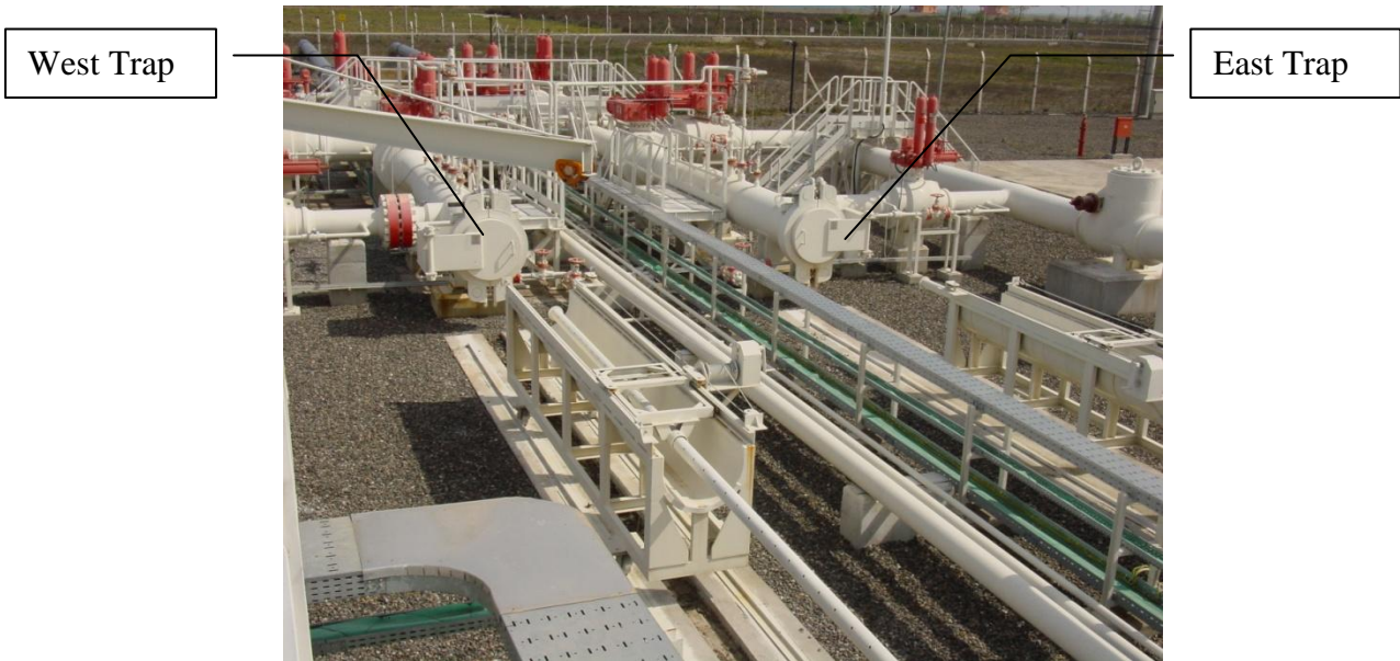
Figure 12- Photograph of the two receive traps in Turkey
