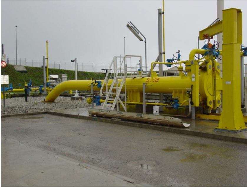
Figure 11- Launch Site in Russia
