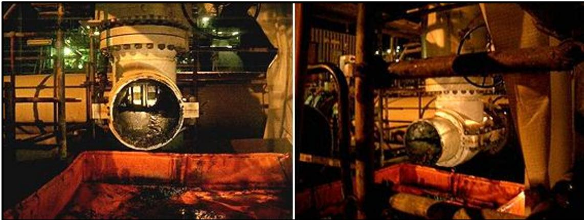
**Figure 11: BISEP™ Isolating Pipeline On-Site with Dead Leg Cut Away**
