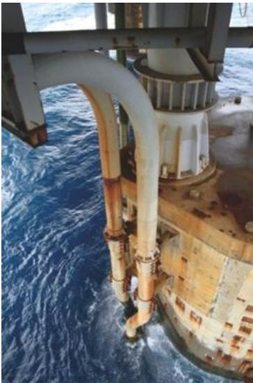
Figure 8: Typical riser configuration incl. splash zone
