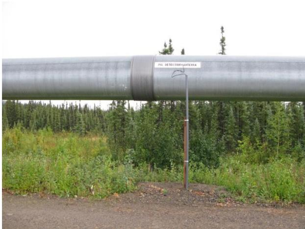
**3004E Antenna attached to the pipe wall at TAPS
