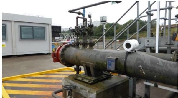
**Magnetic Signaller on a Launcher Barrel**
