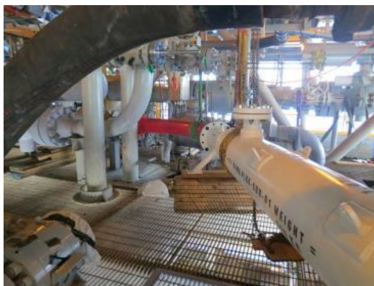
Figure 13: Manufactured PLR installed topside
