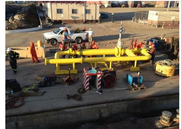
Design enables launching cleaning and MFL pig without intermediate spool recovery.
