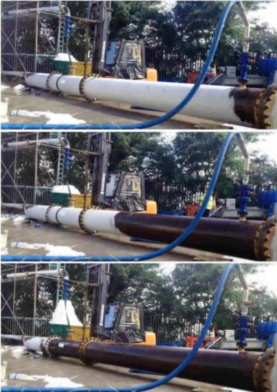
Figure 3 Ice pigging was performed on a dual diameter 24" to 8" steel pipe. The ice and push-water were inserted through a 2 1/2" hose connected to a 2" inlet. Frozen condensation on the pipe shows the progress of the ice plug through the constriction.
