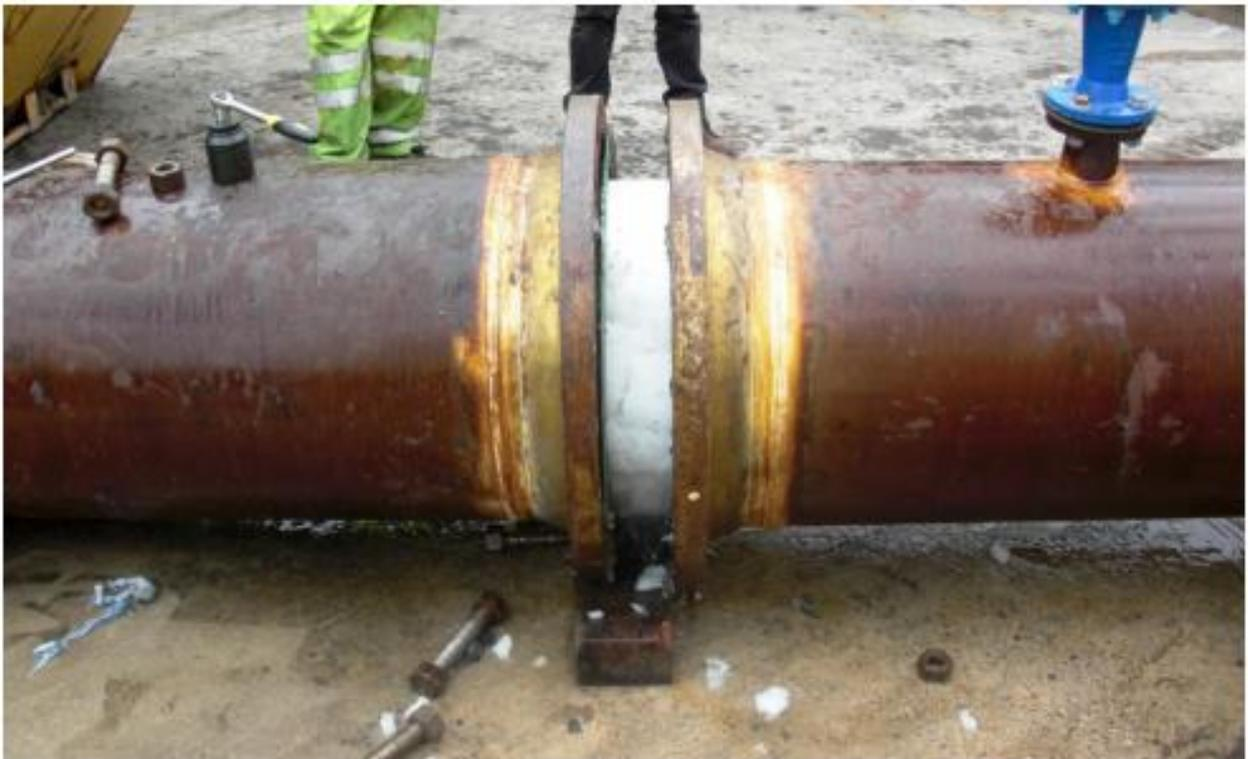
Figure 5 A compressed ice pig holds its shape as the pipe is opened up for inspection.
